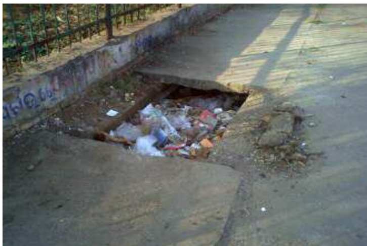
Choked storm water drain with solid waste
