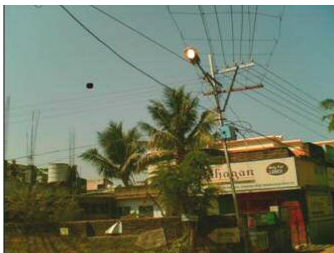
Day-Time Glowing of Streetlights - Poor Energy Management
