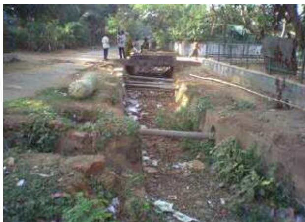
A view of an open drain running across one of the roads located in the CBD
