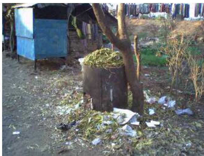
Ill-designed temporary waste storage point with inadequate capacity
